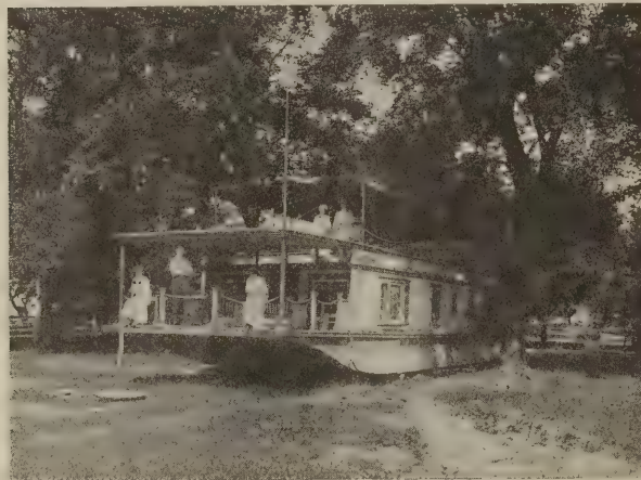
The house boat pulled up on the lawn, ready for remodeling
